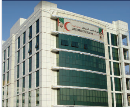
Red Crescent Authority, Baniyas, Dubai AeroSound® LXF
