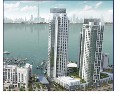
Dubai Creek Harbour Development, Dubai AeroSound® SF
