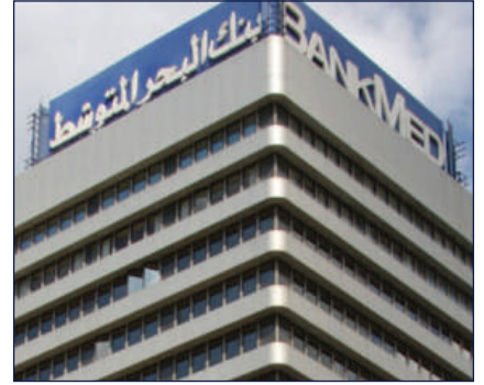
BankMed HQ, Lebanon AeroSound® LX
